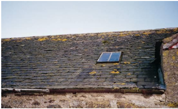
Figure 3 Macduff slate is very durable and is still in use over 150 years after production ceased.
