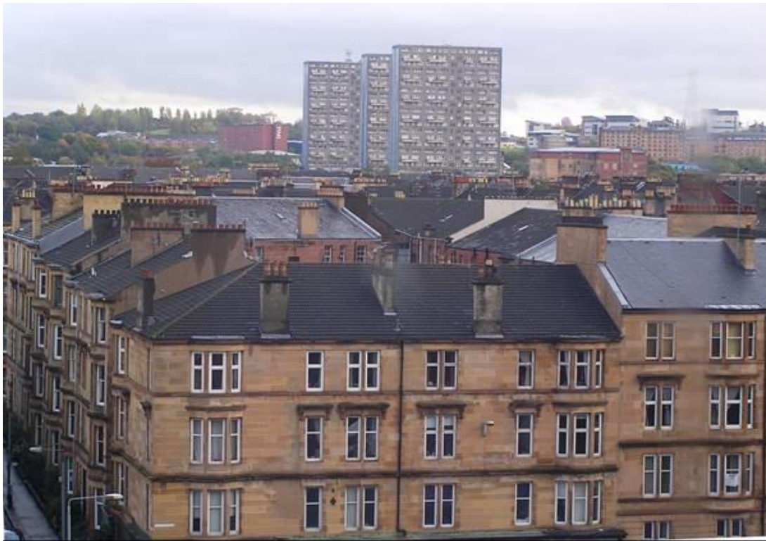
Figure 8 Traditional Scottish slates in this Glasgow tenement have been replaced with Spanish slates and concrete tiles
