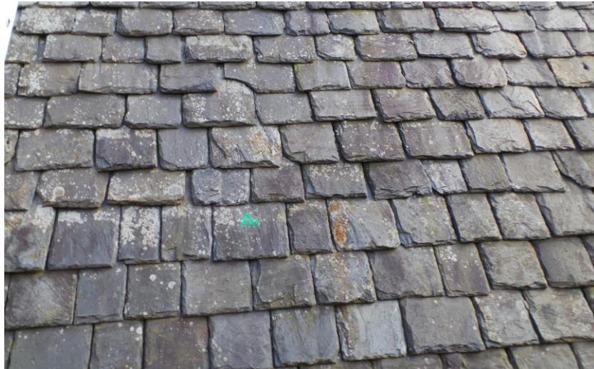
Figure 2 Scottish slates are thicker and more irregular than other non-Scottish slates.
