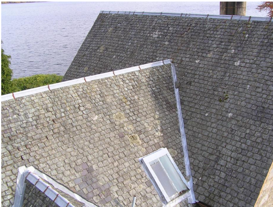
Figure 4 Highland Boundary slate on the Royal Cottage by the shores of Loch Katrine has reached the end of its service life and needs to be replaced.
