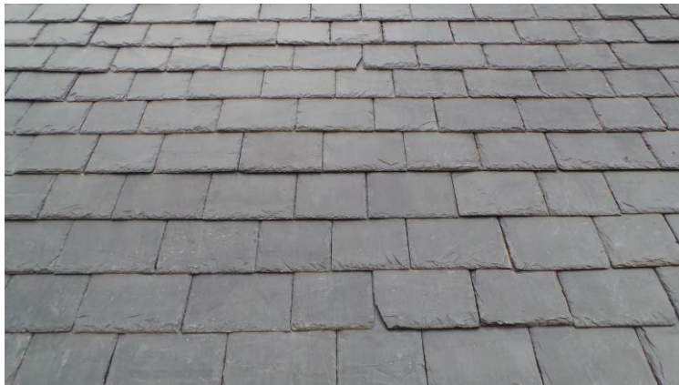
Figure 9b Augustine United Church has been re-slatted with SIGA 120, produced in a range of sizes to replicate the randomness of the original Scottish slate.
