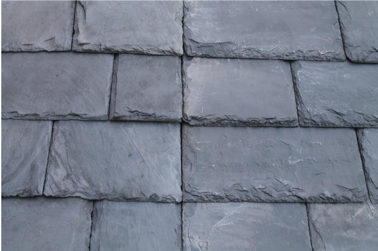
Figure 10 SIGA 120 slates on the right are visually indistinguishable from reclaimed Scottish, probably Ballachulish on the left of this test panel
