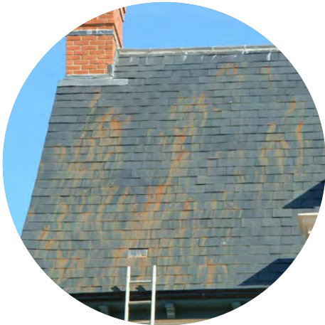
Above: An example of a roof covered in T2 or badly sourced slate
